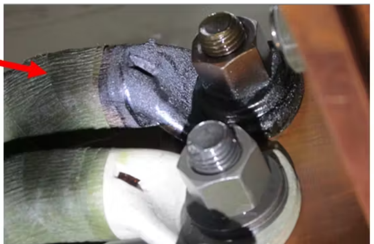
Figure 1. Hydrogen was generated in the transformer oil because of overheating on a low-voltage bushing connection owing to a loose nut on a 500-MVA generator step-up transformer. A hydrogen monitor alerted the owner to the problem. The transformer was repaired on-site.
