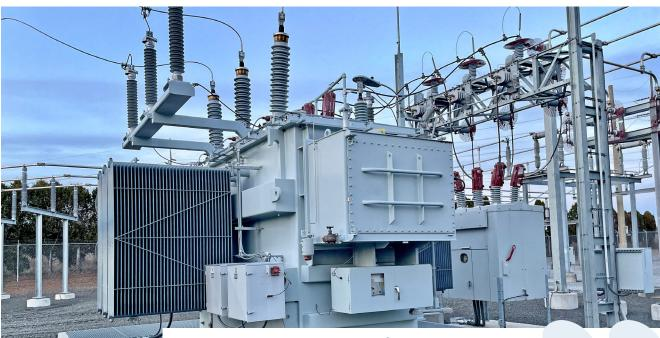
Unplanned loads on transformers in locations with charging vehicles can shorten transformer life due to the stress that includes harmonics induced by charger electronics
