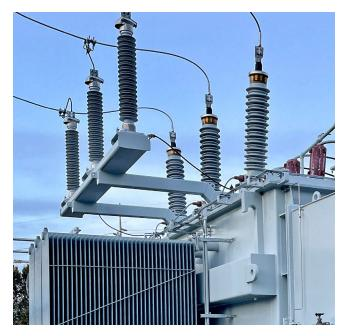
The most widely used tool to understand the health of the transformer is to measure the dissolved gases in the transformer insulating fluid. When thermal and or arcing faults occur inside the transformer, the insulating fluid and solid insulation degrade and form gases in the fluid. By analyzing these gases, the health of the transformer can be assessed. The value of online monitoring solutions is that they alert operators when fault gas levels are increasing inside the transformer.
